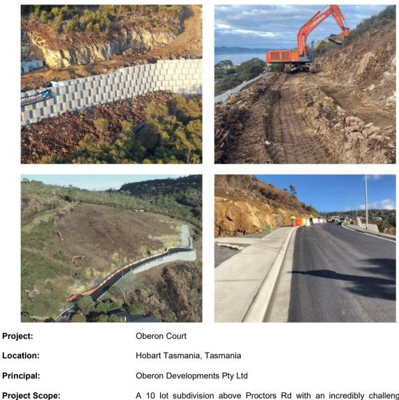
A 10 lot subdivision above Proctors Rd with an incredibly challenging environment, working around a cliff face and on steep slippery terrain. Over 350 mass blocks and 750m3 of no fines concrete was used in the construction of the retaining wall.
